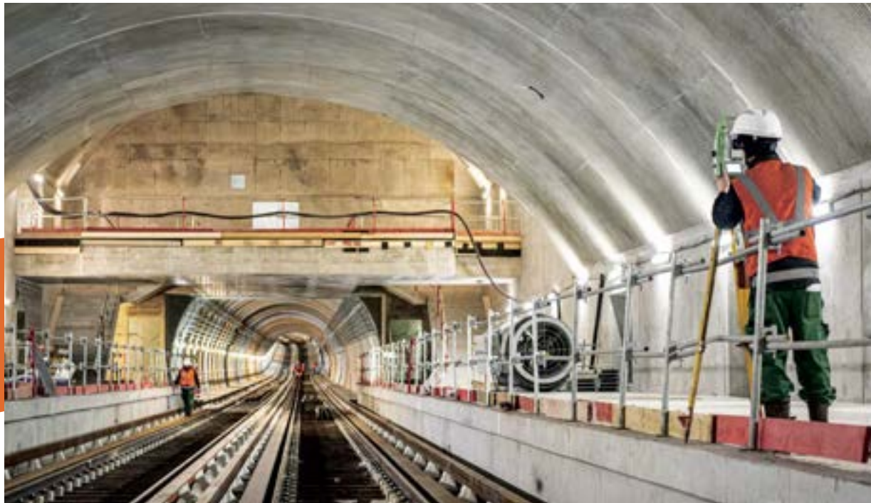
Metro line 4 extension work site.
