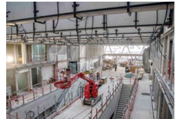
Construction of L'Haj-les-Roses station on metro line 14.
