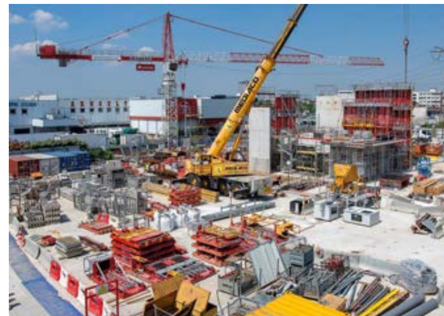
Metro line 14 southern extension work site.
