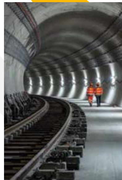
Metro line 14 extension works.
