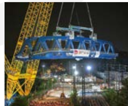
Replacement of the Chartres and Gallardon bridges.
