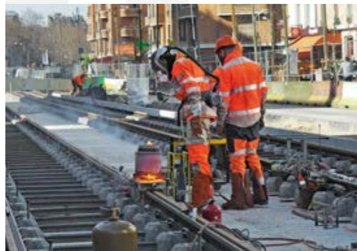
Tram line T3b extension work site.
