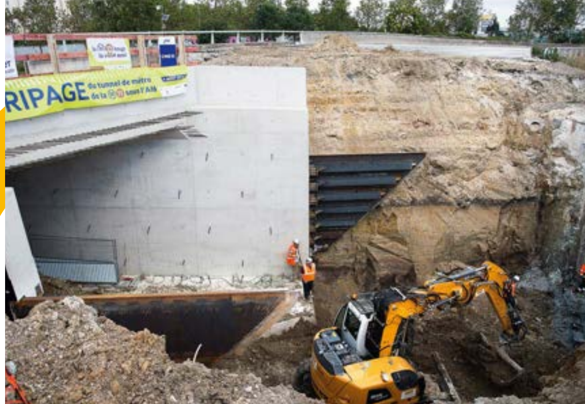
Metro line 11 tunnel excavation and sliding works under national highway A86.
